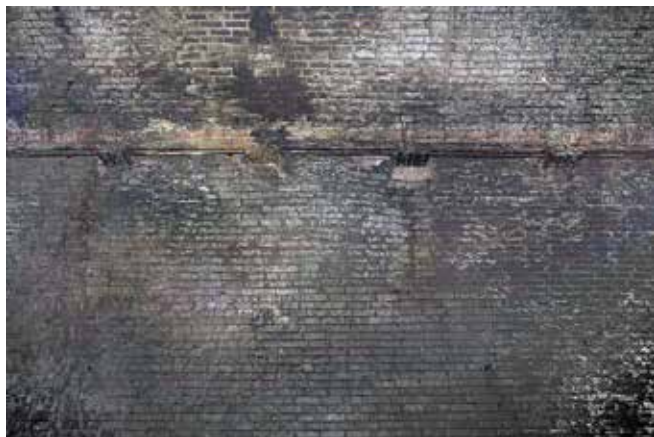
Side wall of tunnel interior
